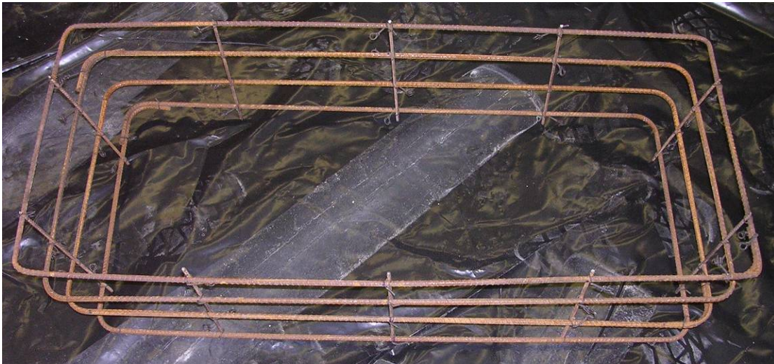
Figure 4.17: Reinforcing Cage for Concrete Jacket Repair
