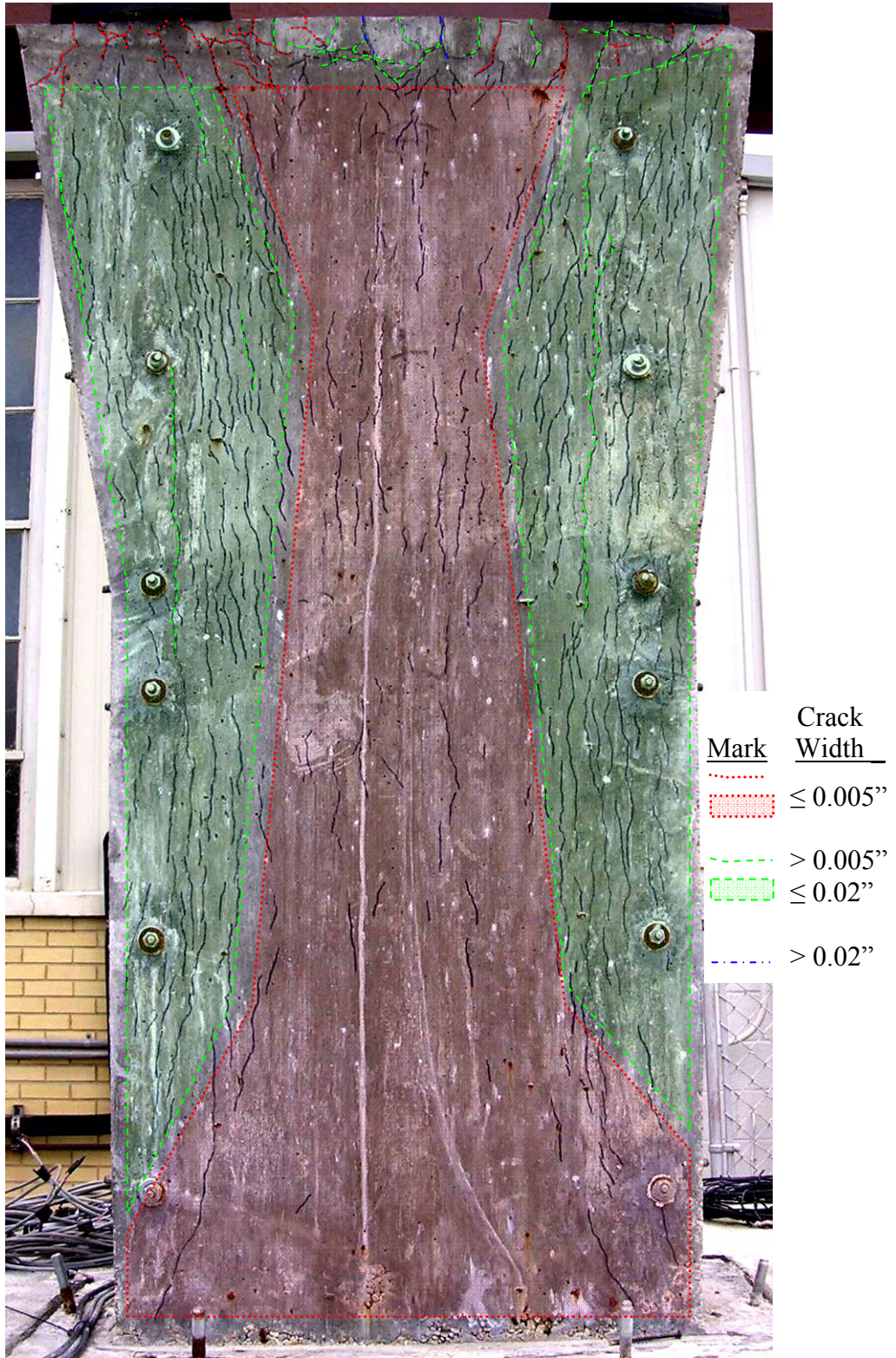
Figure 6.25: Column A West Face April 2008 (cracks marked in blue)
