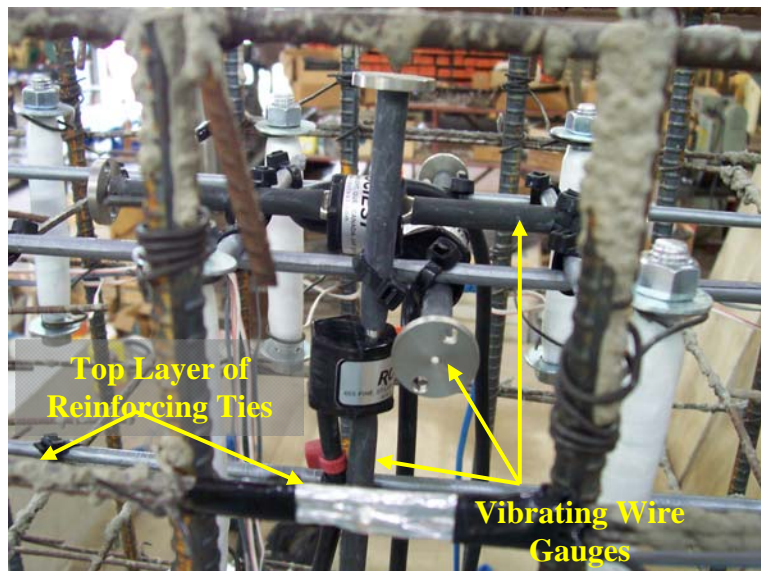
Figure 6.22: Vibrating Wire Gauges in Reinforcing Cage
