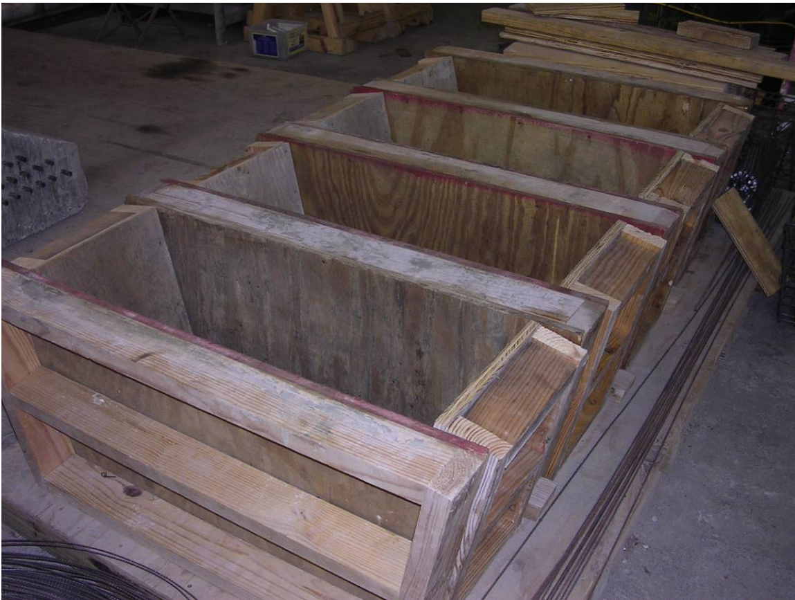
Figure 4.2: Formwork for Bearing Specimens
