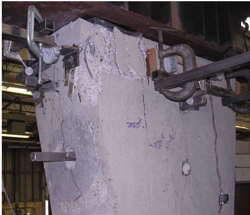
Figure 5.29: Laboratory Failure of Column with an Initial Crack 0.048-inch Width
