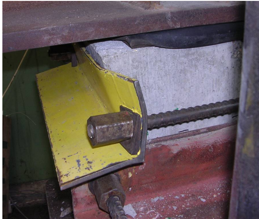
Figure 7.79: Failure of Angle on Post-tensioned #1 Specimen
