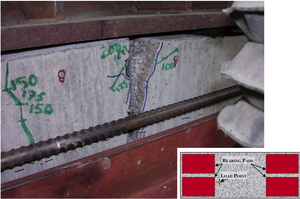
Figure 7.78: Center Crack Widens in Post-tensioned #1 Specimen
