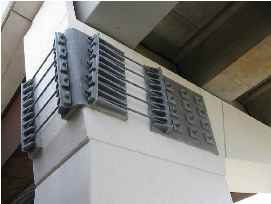
Figure 2.28: Column Capital Repaired with Post-Tensioning 94
