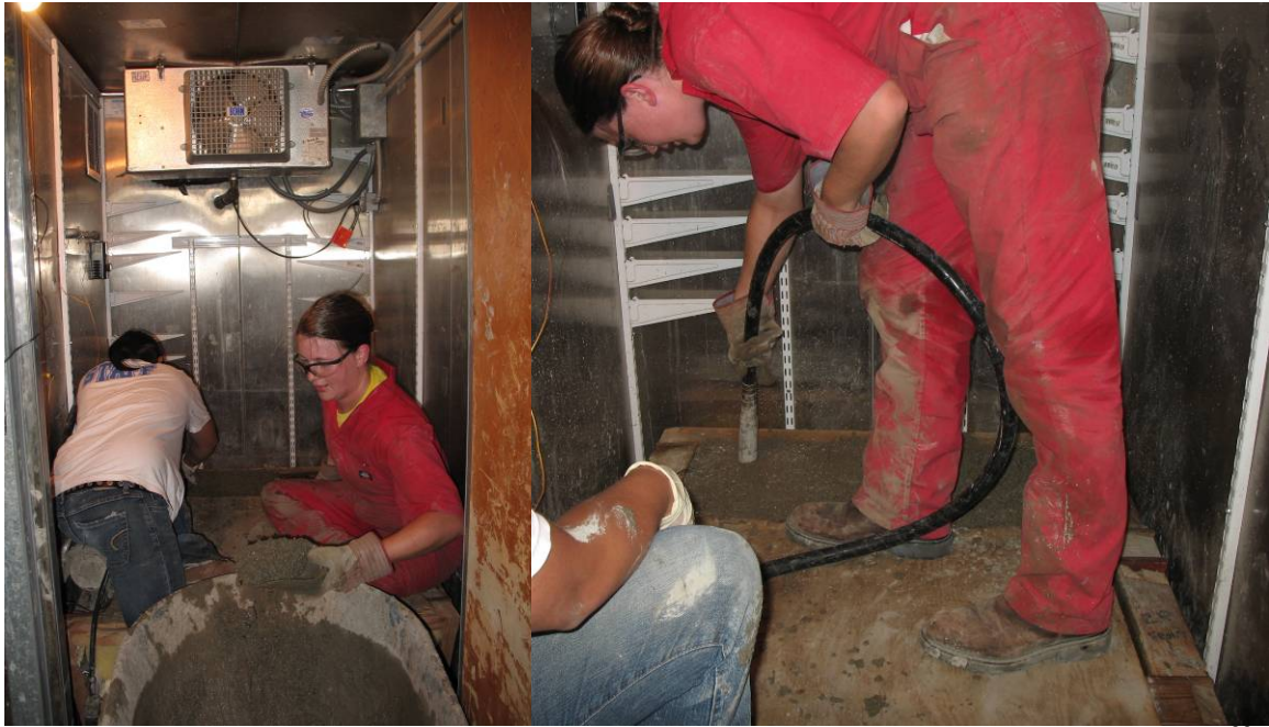
Figure 4.5: Placing concrete in a Walk-in Oven (Left), Vibrating Specimen (Right) 99
