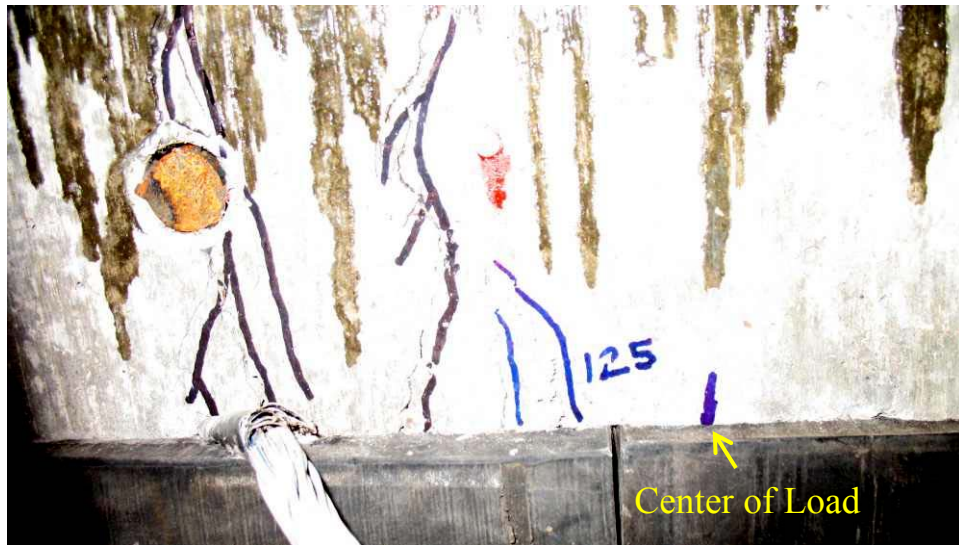
Figure 7.64: Initial Cracking in FRP #2 Specimen
