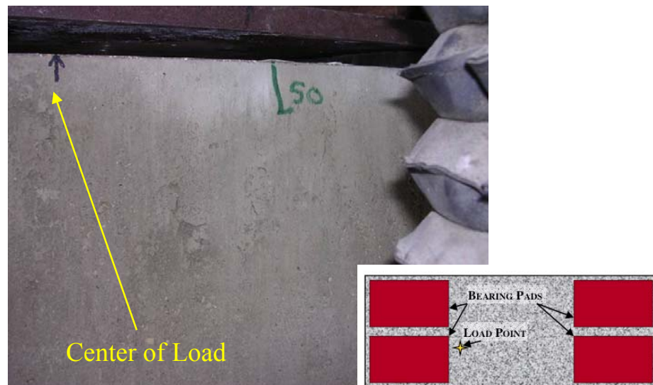
Figure 7.98: Initial Cracking in Concrete Jacket #1 Specimen
