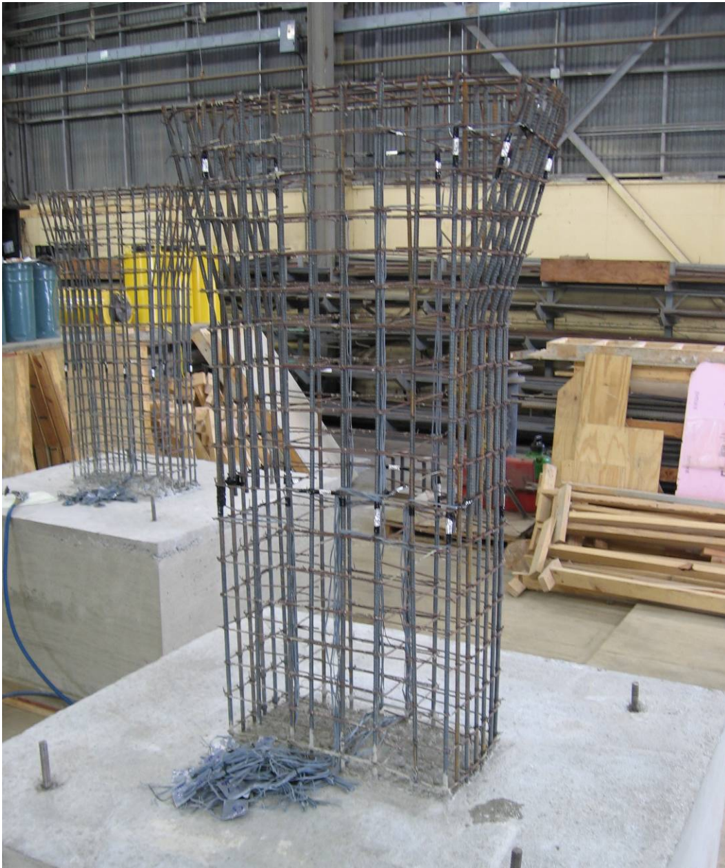
Figure 3.6: Reinforcing Cages used for ASR/DEF Columns
