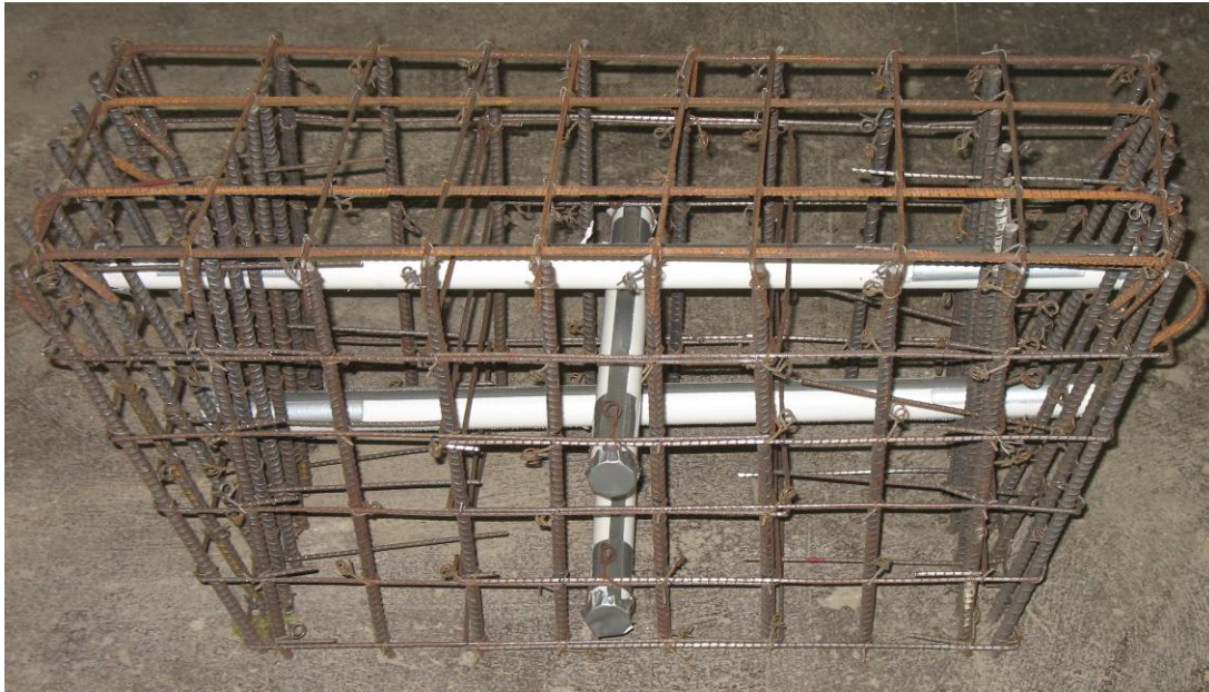
Figure 4.3: PVC Pipes in Reinforcing Cage
