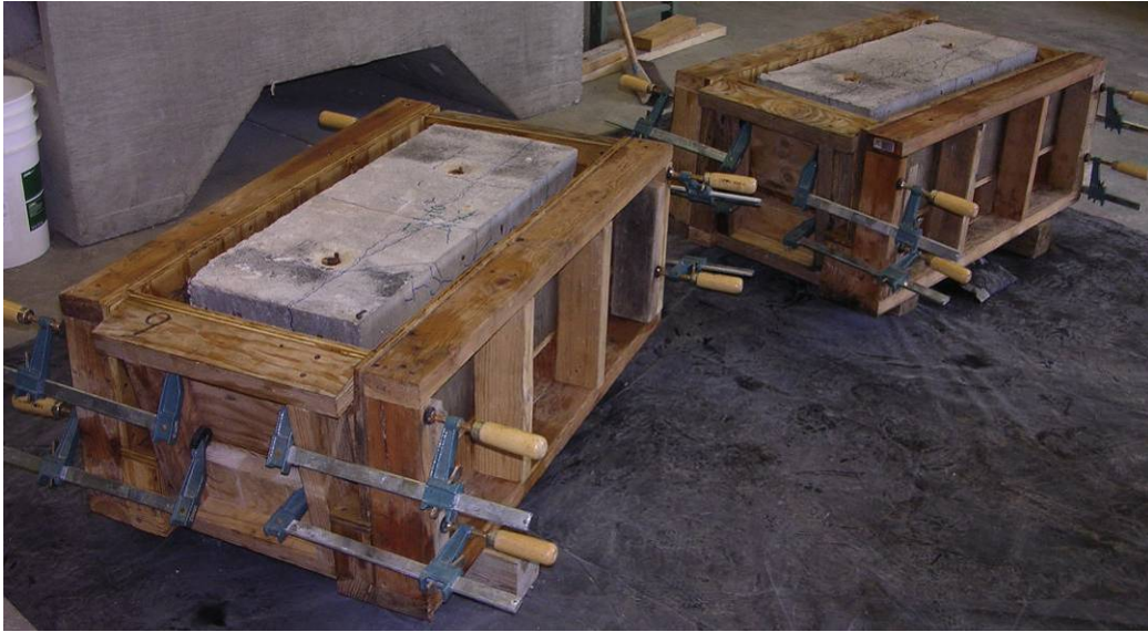
Figure 4.18: Formwork Set Up for Placing Concrete
