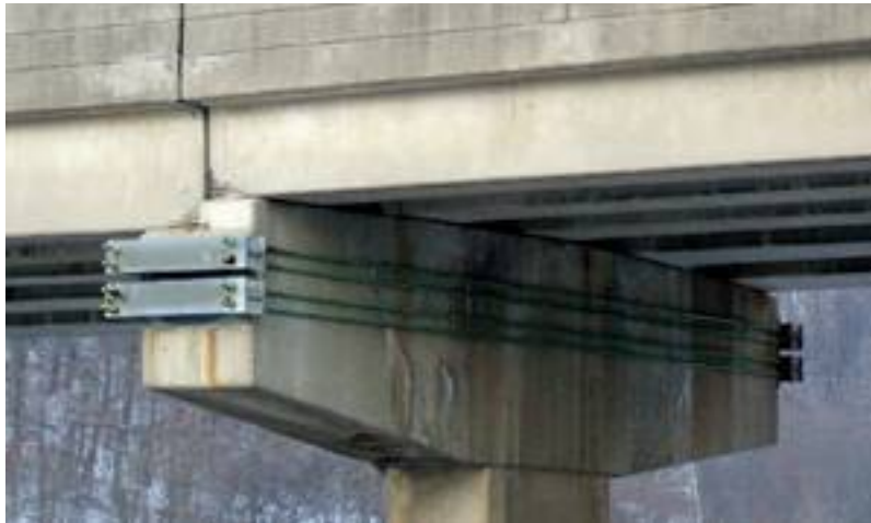
Figure 2.29: Post-tensioning Used for Temporary Repair 90
