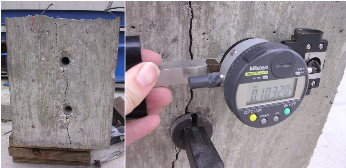
Figure 4.15: Damaged Specimen (Left), Measuring the Crack Width (Right)
