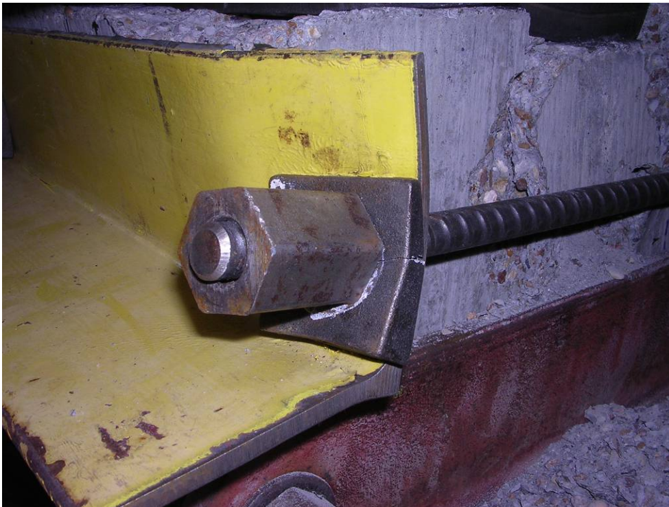
Figure 7.90: Washer Failure of Post-tensioned #2 Specimen
