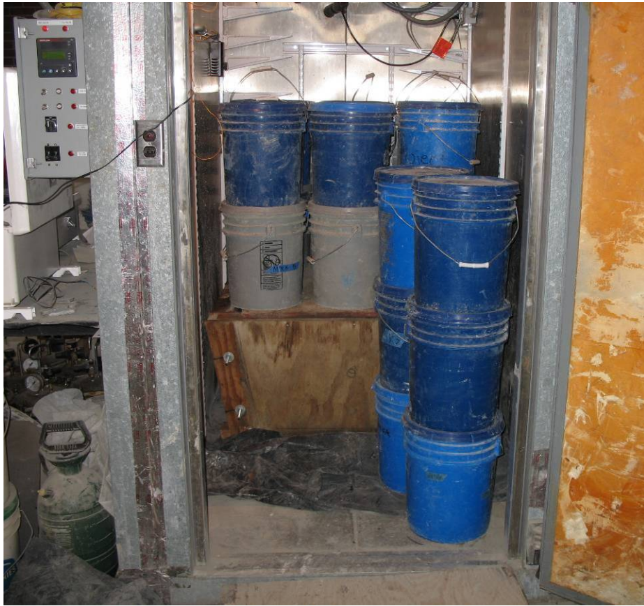
Figure 4.4: Formwork, Reinforcing Cage, and Materials in Oven to Preheat
