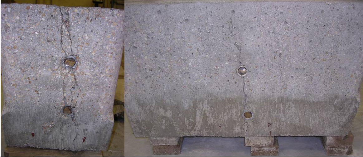
Figure 4.25: Prepared Concrete Surfaces for FRP Application
