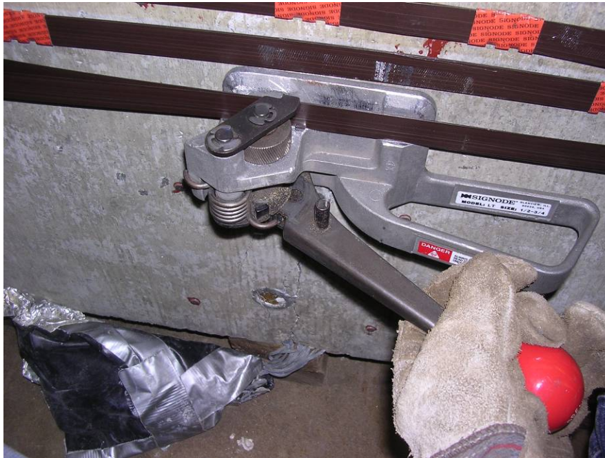
Figure 4.23: Tightening Packing Strap using Hand Tools
