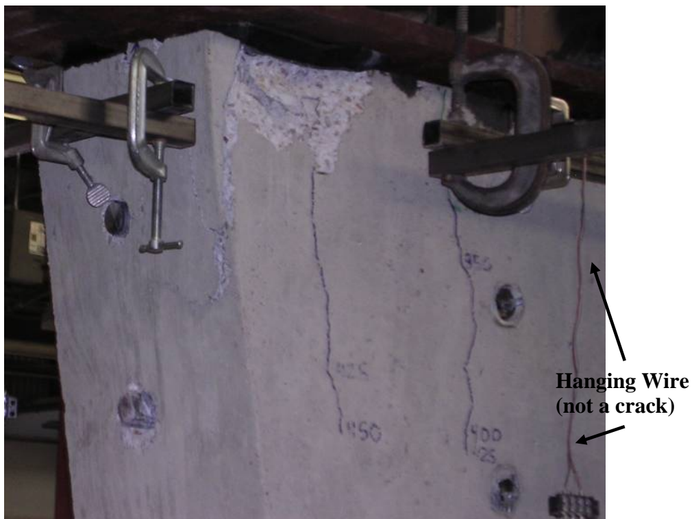
Figure 5.13: Cracking Pattern at Failure for Kapitan's Control Column
