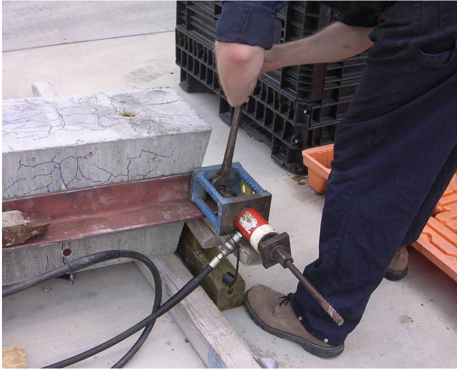
Figure 4.20: Tightening the Post-Tensioning Nut
