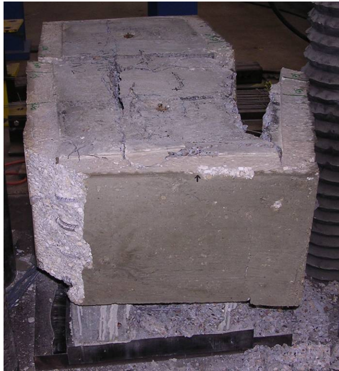
Figure 7.115: Concrete Jacket #2 Specimen Damage
